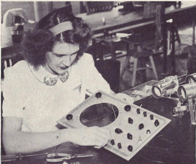
WITH THE PANEL COMPLETED, Katheryn Elensky inspects each part to see that it is in working order. This is one of many checks given a test instrument before it is shipped.
