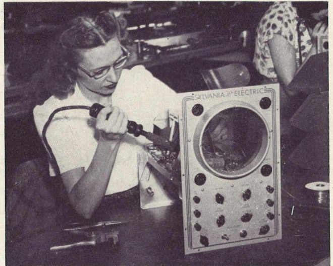
NOW MORE PARTS are added to already complicated chassis. Louise Reeder handles the soldering iron with skill.
